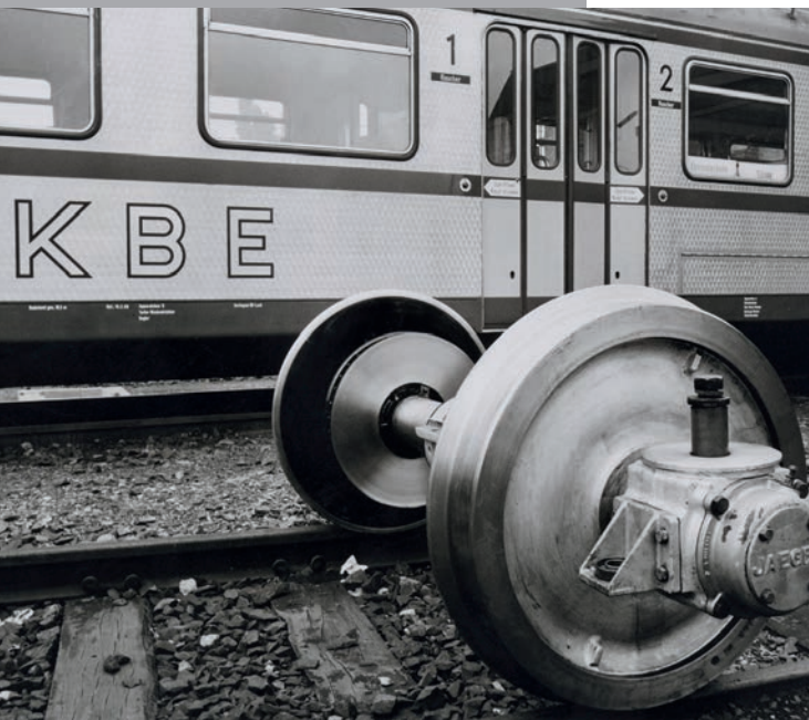
Aluminium-steel wheelset for the Köln-Bonner Eisenbahn (1960s)
